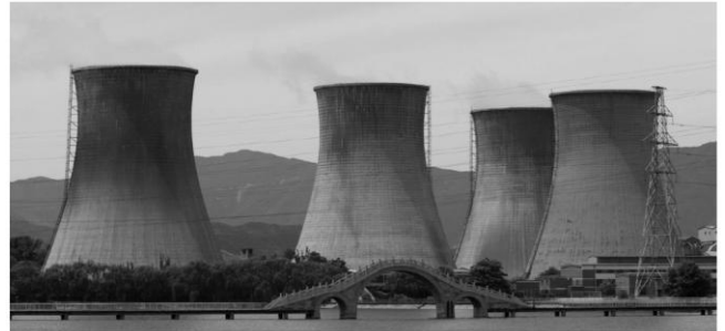
Fig.1. Group of Natural Draught Cooling Towers
