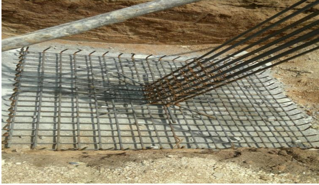
Fig.5. Screen 3.1: Steel Reinforcing Bars on Site
