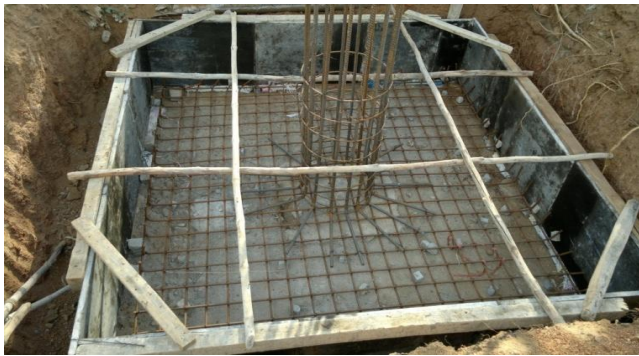
Fig.6. Screen 3.2: Centering and Formwork on Site During Execution
