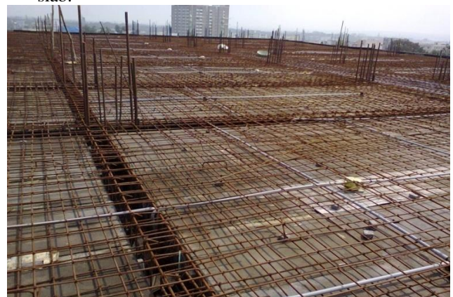
Fig.9. Screen 4.2: One Way Slab
